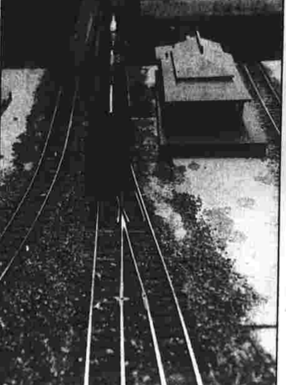
DOWN THE TRACK — The Buff Valley Railroad crosses a bridge.
